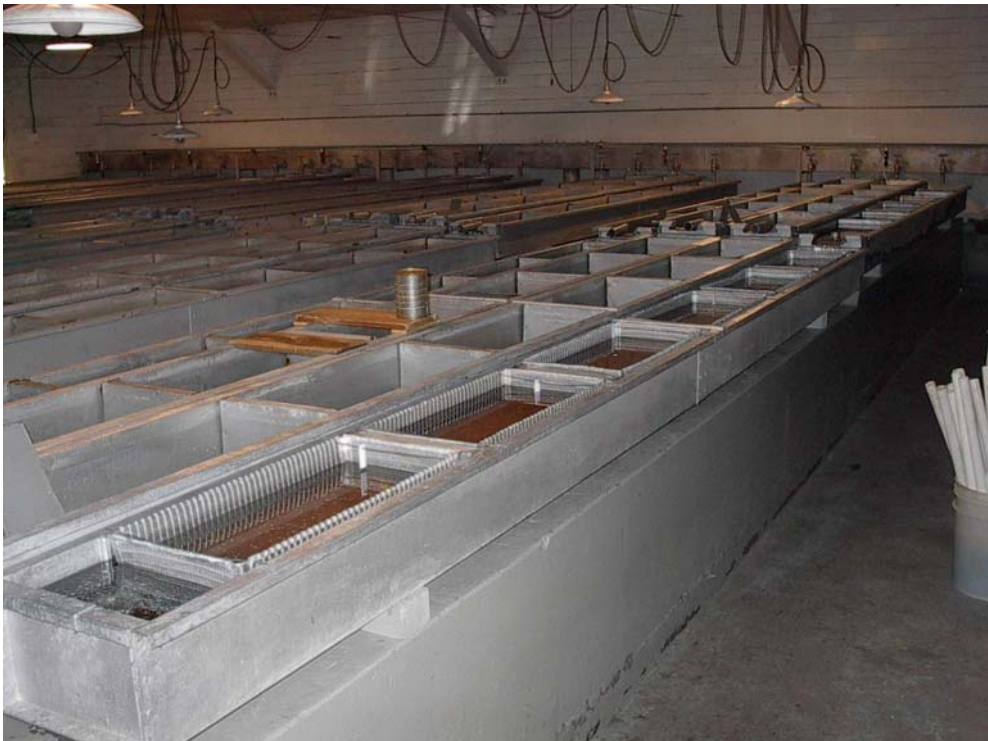
Ford Hatchery (1941) trough and tank room.
