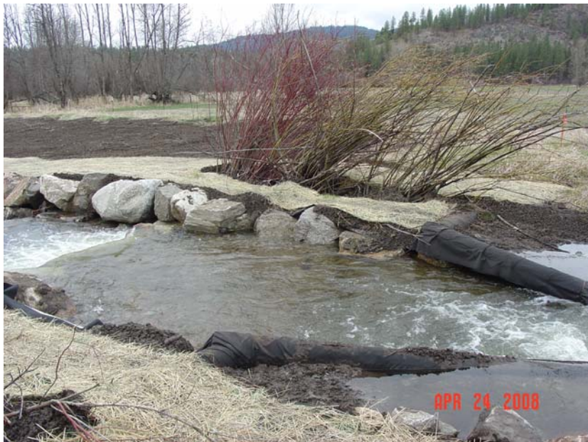
Figure 6. Photo at the head of the structure where k-log structures were placed into the bank to channel flow and limit bank erosion.
